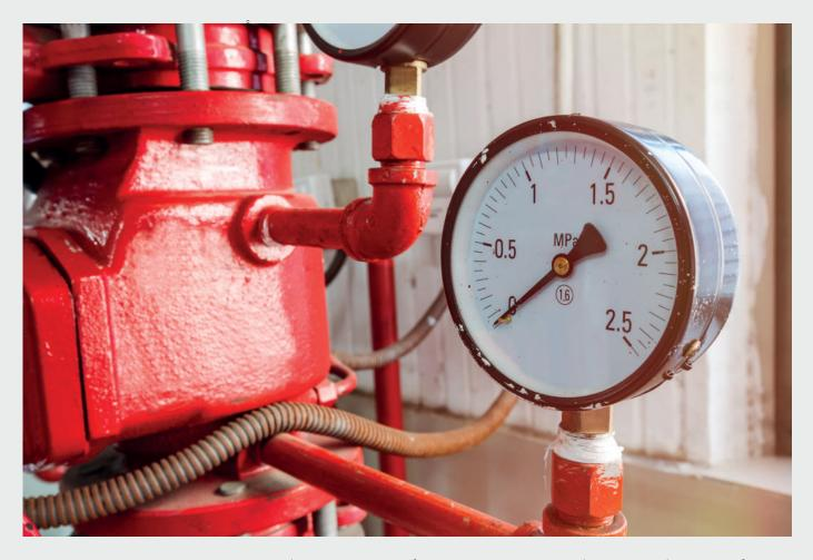
The alarm check valve is a water flow alarm device designed for vertical installation in the main supply to a wet pipe sprinkler system. When a flow of water from the system equals or exceeds that of a single sprinkler, the valve is to actuate a fire alarm.
